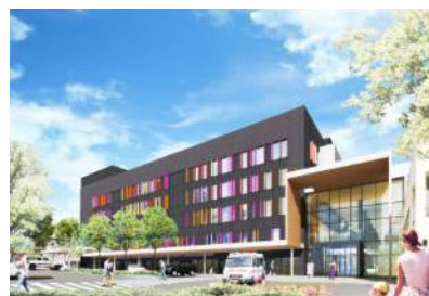
The finished stage 1 BMDH expansion
